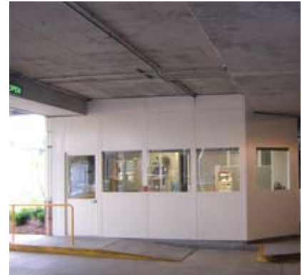
The modular panels used to construct the office inside this hospital parking garage were custom designed to fit under the existing ceiling structure.
